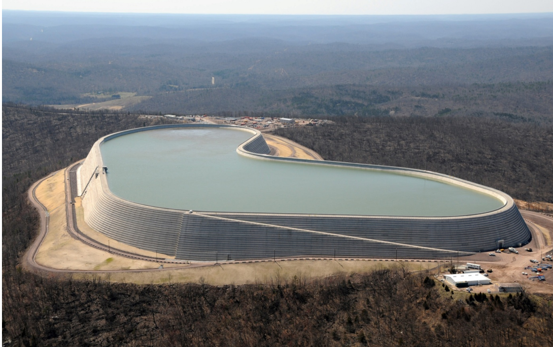
Figure 7-6: PHES upper reservoir (of Taum Sauk PHES in the USA) with a man-made reservoir wall [159].
