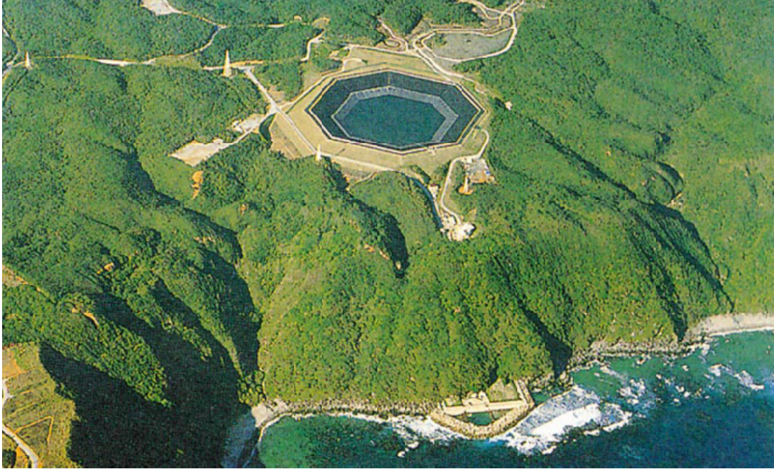
Figure 6-2: Photograph of a pumped hydroelectric storage facility using seawater [92].
